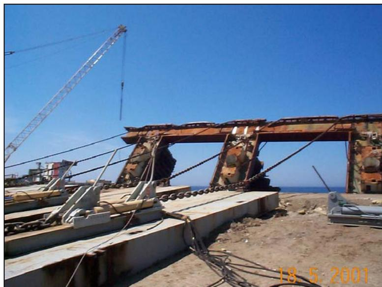
*Figure 9: Fore Part of the Wreck showing chain pullers on shore*
