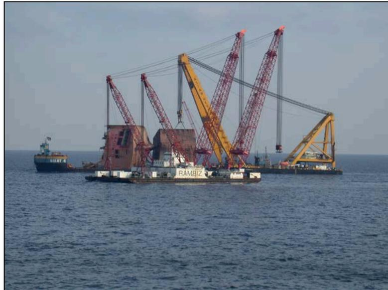
*Figure 4: Sheerlegs lifting the second cut section*
