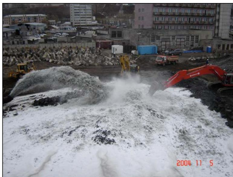
*Figure 11: Rock cuttings being pumped ashore to construct the bund*
